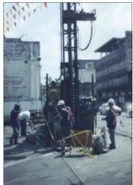
Installation of monitoring wells for ground contaminants survey
