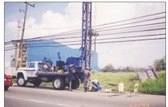
Hollow Stem Auger Drilling for subsurface soil investigation of a pipeline project.
