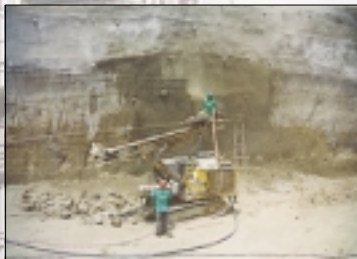
Shotcreting of soil nailed wall in Fort Bonifacio Building Development
