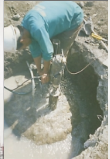
Quality control of jet grouted soilcrete by concrete core extraction. The cores will then be tested in unconfined compression testing apparatus. Average strengths exceed 1000psi in most instances.
