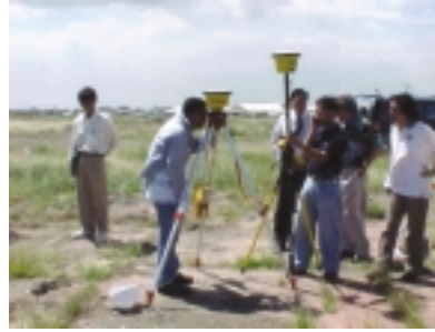
TRIMBLE 4800 Dual Station GPS with RTK Operating Radius of 10 Km being used at NAIA IPT3 Project.
