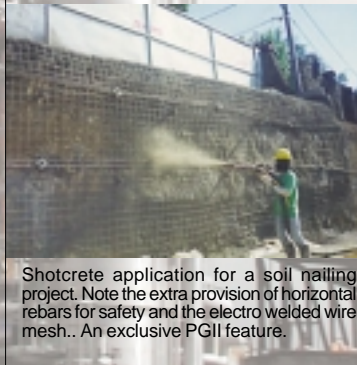
Shotcreting of soil nailed wall in Fort Bonifacio Building Development
