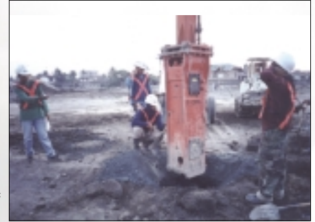
High frequency (500 BPM) hydraulic tamper with bevelled tamper foot.
